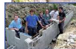
Our group had to overcome heavy constraints on a riverbed based construction site
